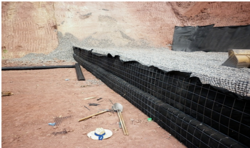
Figure 3. Facing type of the MSE wall
