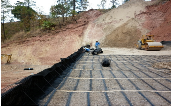
Figure 5. Construction of the first wall (2011)
