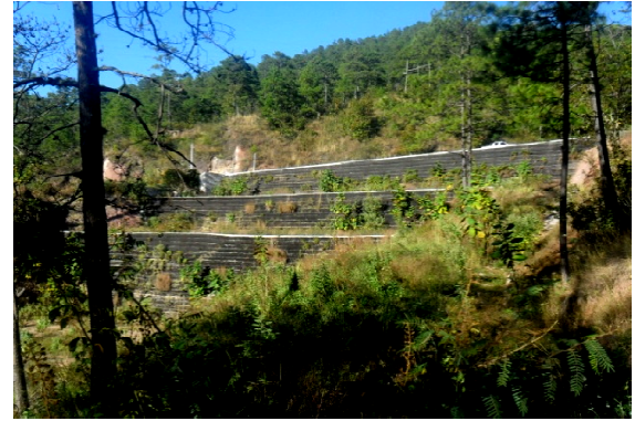
Figure 8. Panoramic 2013's view of the MSE wall constructed in the km 11 of the CA-6 highway
