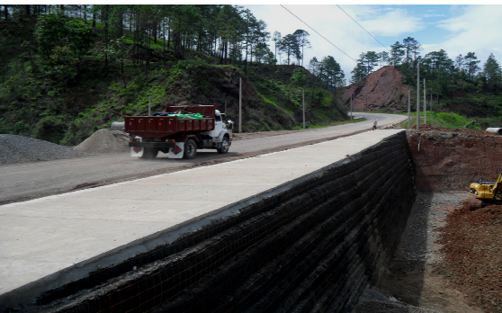
Figure 7. Construction of the third wall (2011)
