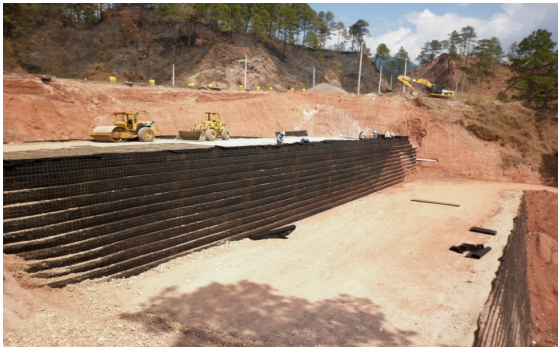
Figure 6. Construction of the second wall (2011)
